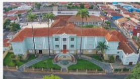
HOSPITAL UNIMED - SANTA CASA
